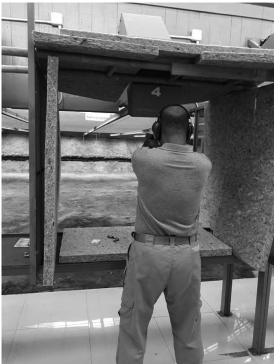
Figure 3 Using 4 square meters of 5 cm. thick recycled polystyrene drinking bottle as sound absorption material.
